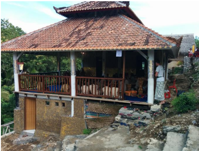
New building in FNPf Nusa Penida
