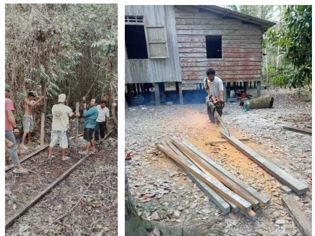
Our staff built the bridge in Jerumbun
